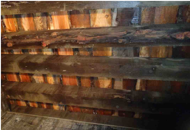
Figure 1-9: Typical deck soffit condition.
