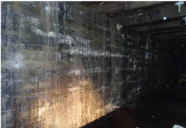
Figure 1-11: Downstream girder exterior face.
