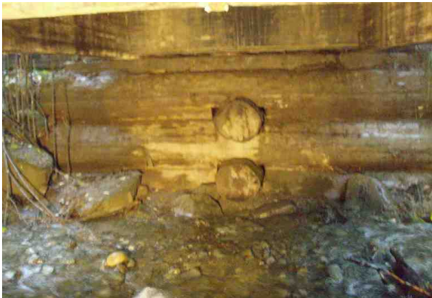
Figure 1-15: Woods end log crib.
