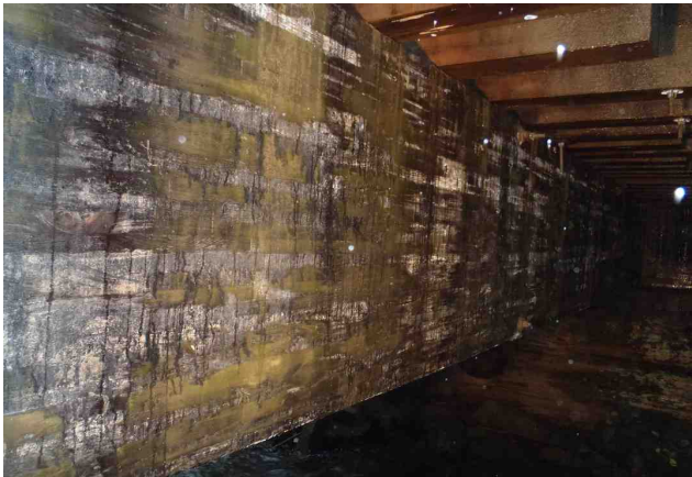
Figure 1-10: Upstream girder exterior face.
