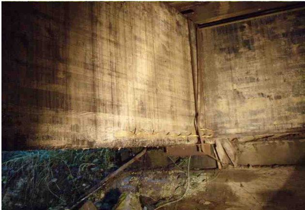
Figure 1-14: Epoxy injection tubes on the interior face of downstream girder near camp end.
