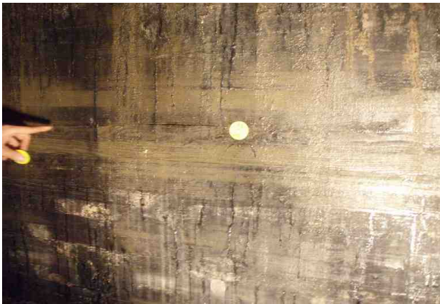
Figure 1-12: New check tagged on downstream girder exterior face.
